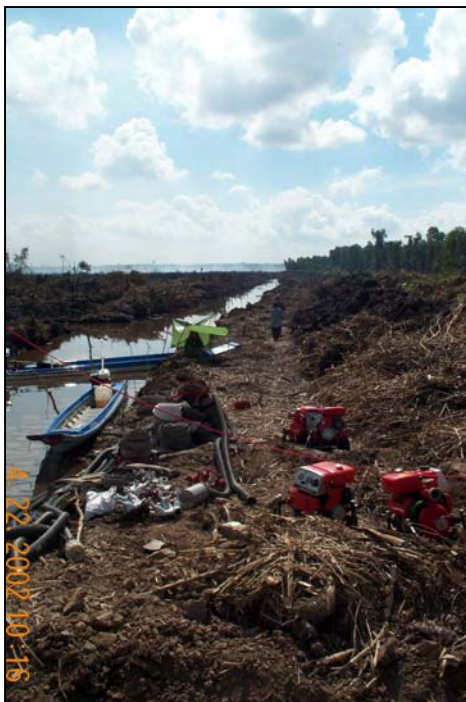
Figure 6. Approximately 15 km of newly constructed canals
